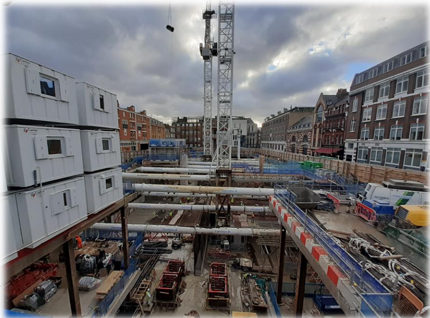
South core construction and commencing ground floor slab
