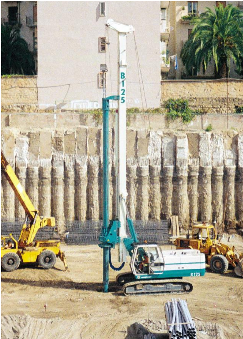
CFA rig for soft piles
