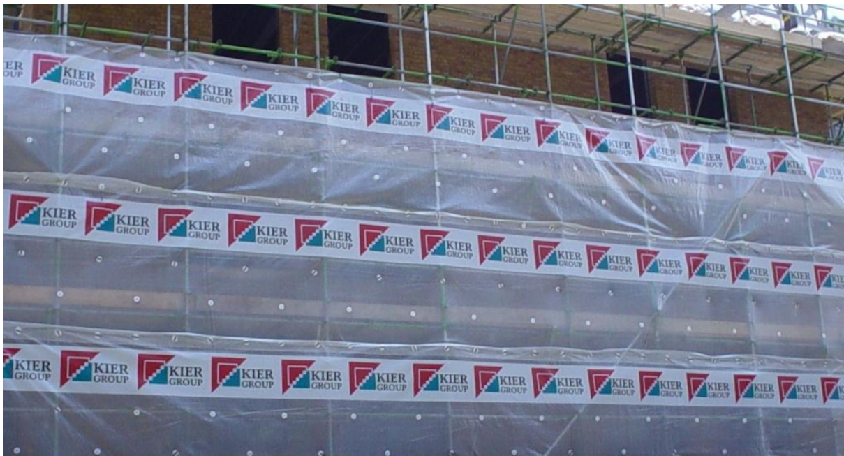
Example of a fully enclosed scaffold with monoflex
